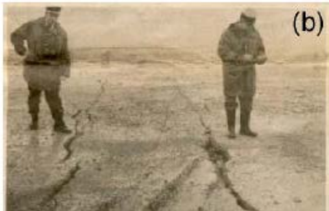
Cracks in the Airport runway related to the landslide event
